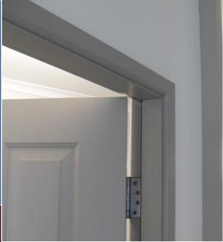
The door frame shown here features a shadow line rather than architraves. This again is identical to the windows treatment available in both a flush and sunken finish.
