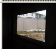
5. Temporarily fit the window. Two screws in the head are sufficient. Use the screws you normally would to fit the window.
